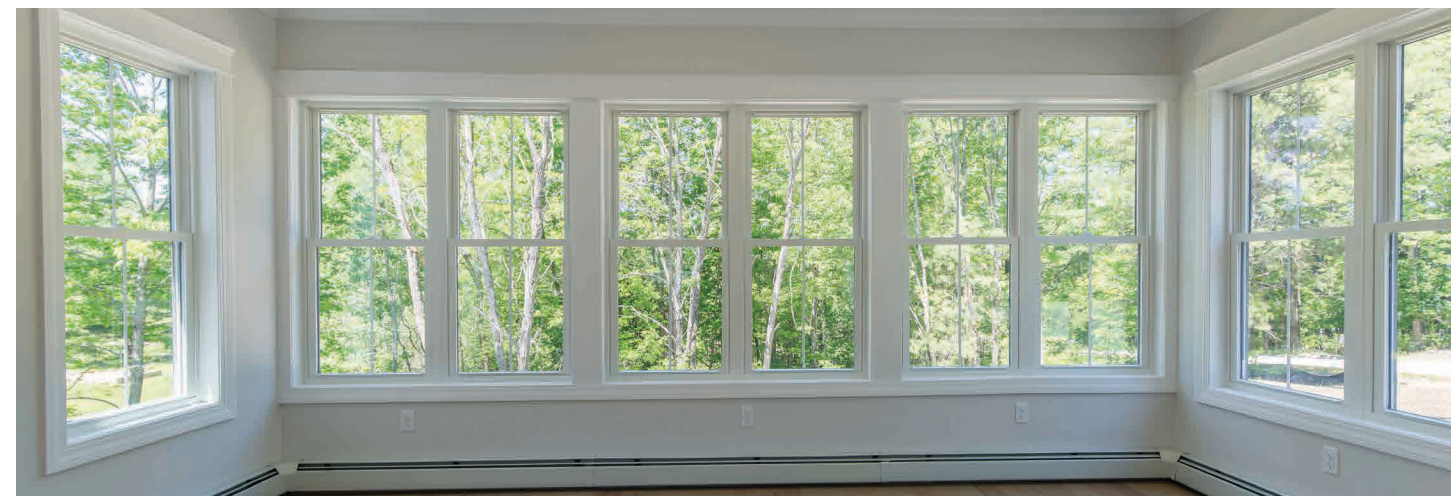
Photo provided by Robie Exteriors - 2020
